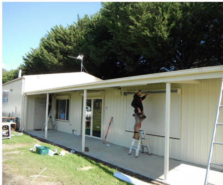
Pictured: Security Roller Shutter Installation
